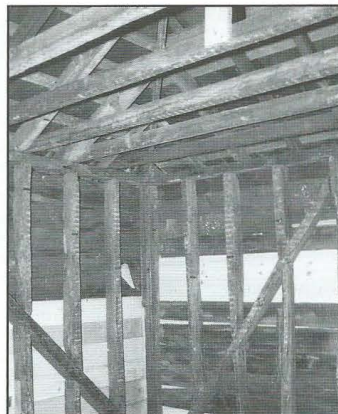
Interior view during reconstruction showing the locally sourced hardwood studs.
