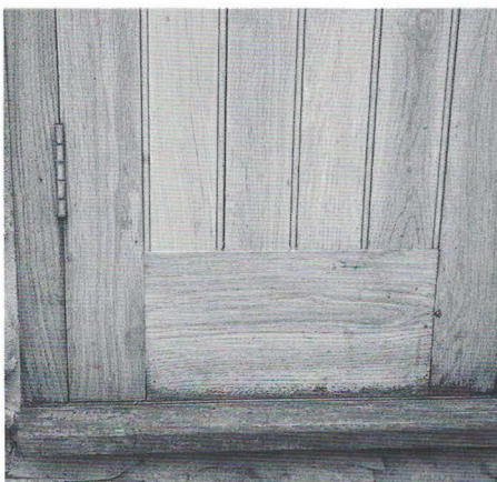
Water Penetration and staining through un-sealed end grain on bottom edge of door.
