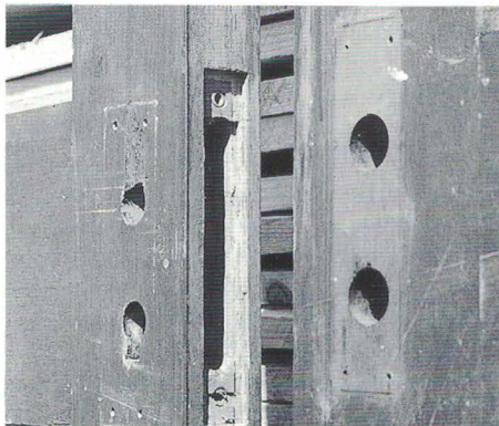
A mortice to receive a lock case which has all but destroyed the integrity of the joint between the stile and middle rail.
