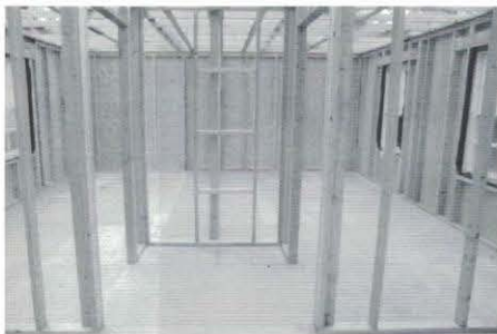
Internal and external timber stud framing in a platform frame construction
