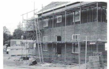
A timber frame, brick clad, house nearing completion of the external walls and roof
