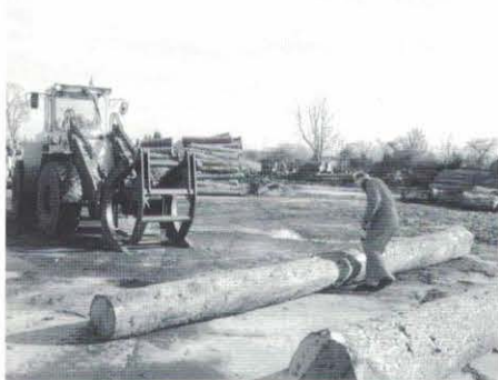
Selecting and measuring individual larch logs for heavy construction beams
