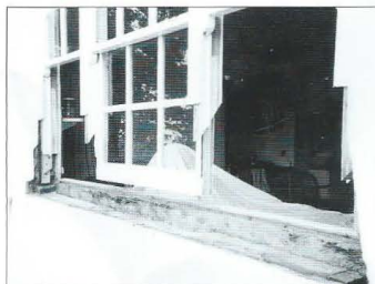
All rotten wood removed, stiles, mullions and sill cut away at angles to take new timber repair
