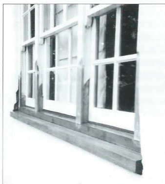
Repair complete. New sill, mullions and stiles repaired with quality softwood. Acute cuts to splices facilitate successful outcome almost end grain fixing.
