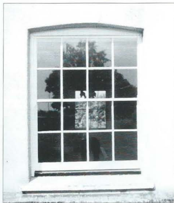
Historic window (box frame ©1790 Sashes after 1850) which needed extensive repairs to the sill and lower frame. The picture shows the completed repair and the window restored to full working order.
