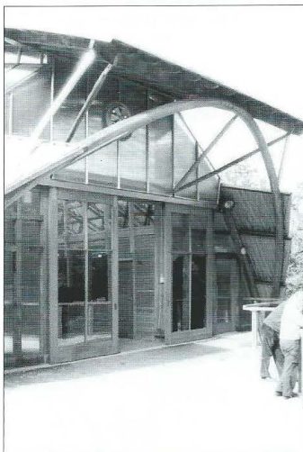
The main entrance to the gridshell showing the specially constructed glulam arch
