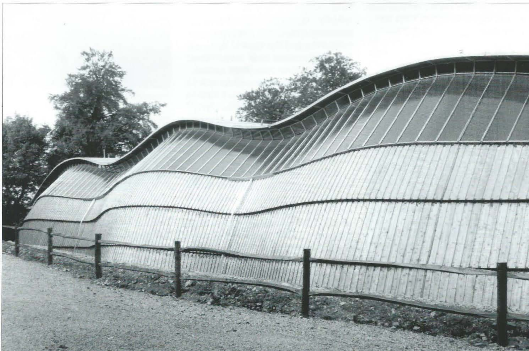
An external view of the gridshell showing the British grown western red cedar boarding
