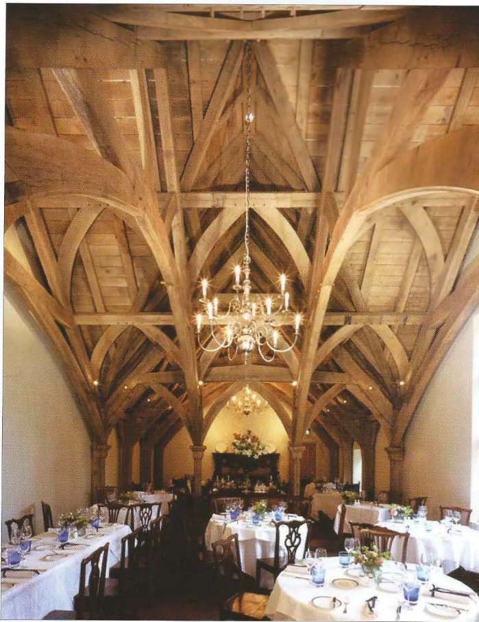
View of the complex sling-braced oak trusses above the Great Fosters Hotel restaurant area
