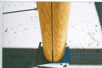
Detail of the base of an arcade post showing the flitch plate ground connection and the stress-relieving saw cut
