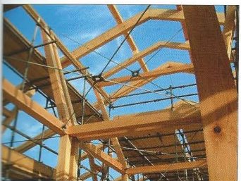
The light-well formed in the upper part of the roof structure.
