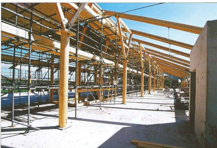
General view of the interior of the structure showing the arcade posts and principal rafters
