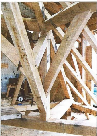
The complex corner design as seen from the interior of the structure showing the individually cut, shaped and jointed components
