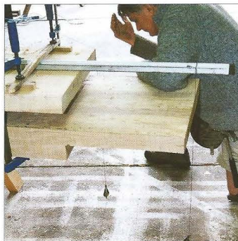
Centering the beam with the datum line on the floor using a plumb bob
