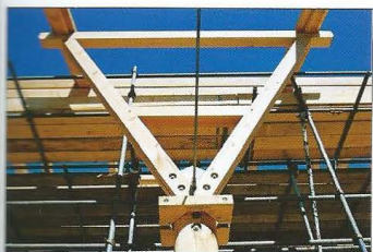
The saddle truss arrangement capping the arcade post and supporting a pair of principal rafters
