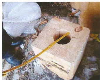
Centre boring in Norway, size of hole is critical
