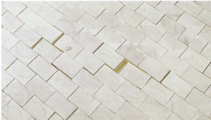
Woodblock floor suffering from severe shrinkage. (It had been sawn "green" but installed in a library where the equilibrium moisture content was about 12%. Need we say more?)
