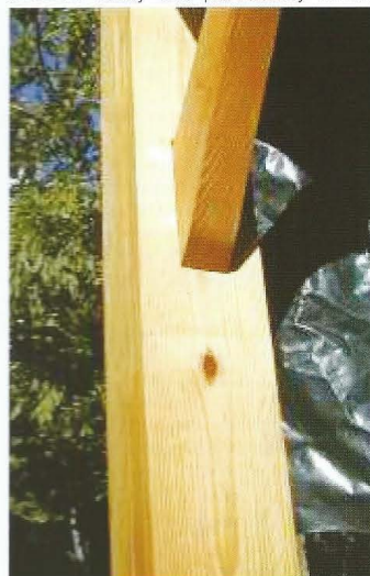
The face side of the same post showing a 'check-free' surface
