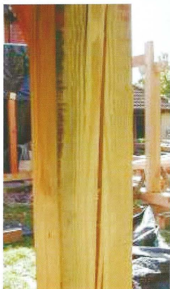
Large natural drying checks on the rear of a post
