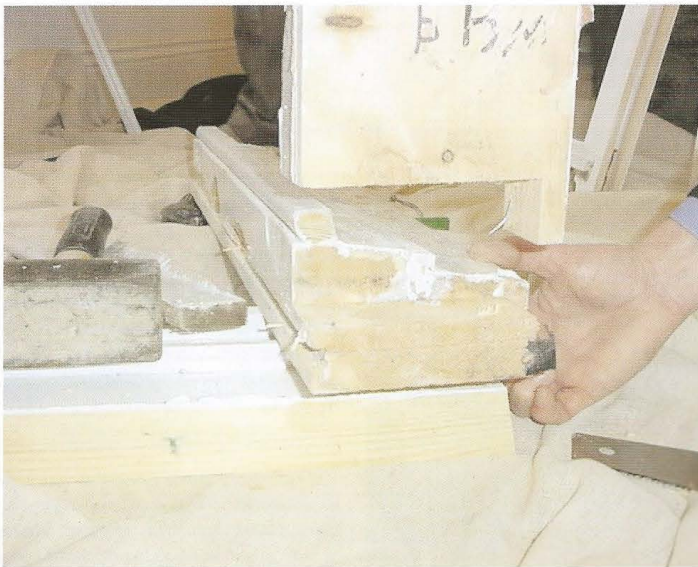
A sash window joint which was dismantled to prove that no sealing or gluing of the timber had taken place at the time of manufacture. (In service, the window was leaking rainwater internally at this crucial joint, which had been formed by "trenching" through the entire cill section.)
