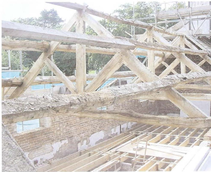
Old barn timbers, intended for structural re-use in situ: but the decision in this case was that there was too much deterioration from insect and fungal attack to warrant any guarantee of future life in the conversion to a new dwelling.
