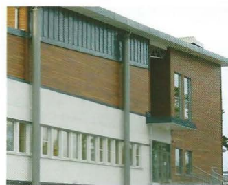
Stora Enso ThermoWood cladding at the Fredrica Bremer school, Stockholm. Pigmented coating applied before installation.
