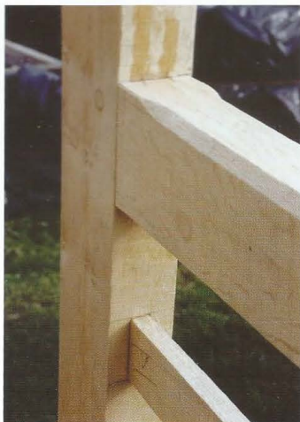
Detail of the pegged joint between top rail and butt post with intermediate rails loose fixed in mortices.
