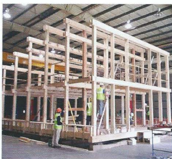
Assembled glulam frame.
