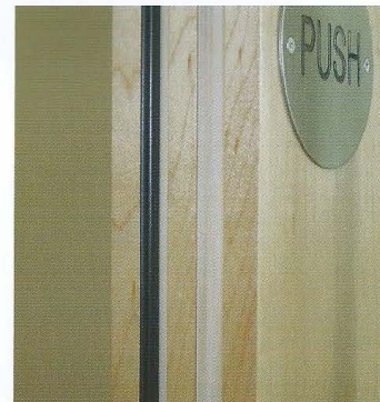
Door edge showing both the intumescent strip (in white) and the smoke seal (in black). Photo D E Woodbridge.
