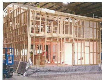
External studwork modules and membrane installation.
