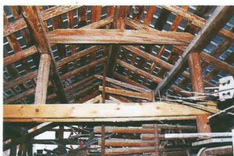
The inserted box frame intended to replace the original roof truss.
