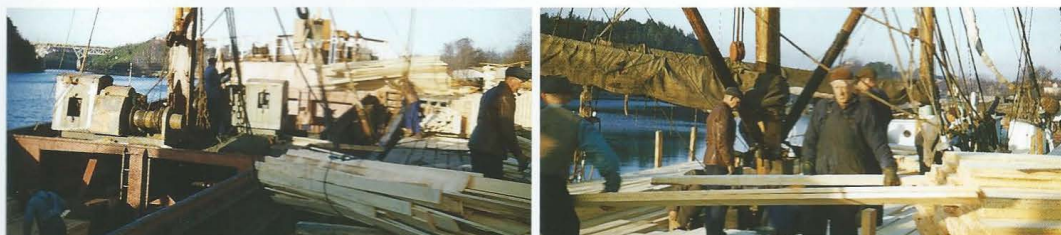
Loading softwood in Sweden in 1956 using the ship's tackle and stowing the timber piece by piece (bottom left)
