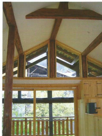
The new roof supports.
